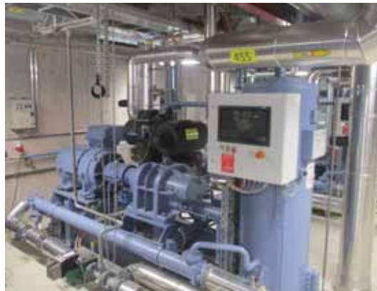
➤ Screw compressor package with GEA Omni control panel
